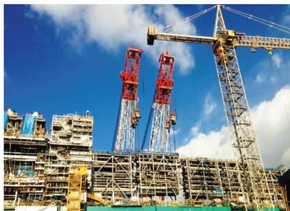
Figure 3: Lifting of the last pipe rack module
