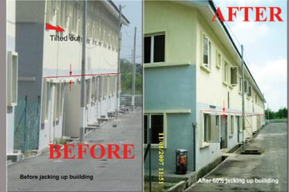
\*Building Settlement tilt correction using Inocative underpinning piling techniques that can be **proof-loaded** and **pre-loaded** to lift up the building and be locked-off permanently. **Pile Driving 20t - 350t WITHOUT KENTLEDGE** using
